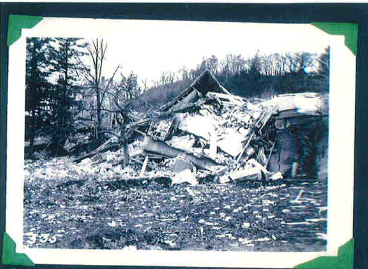
RUINS OF HOUSE DESTROYED BY
