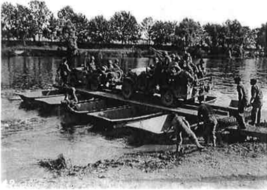
Ferrying Equipment across the Moselle River
