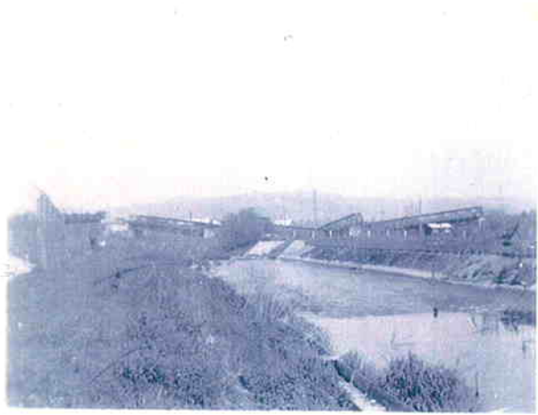
Blown bridge at Braneau, Austria
