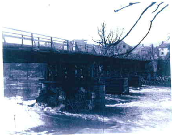
Fixed Bridge, Diekirch
