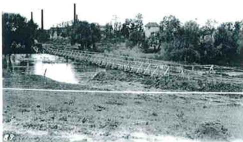
Fixed Bridge at Pont a Moussen
