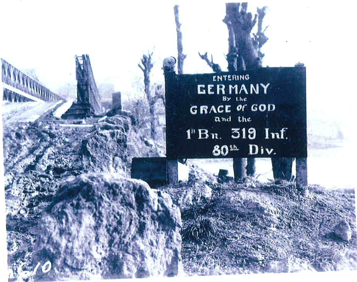
Approach to Bridge Wallendorf, Germany
