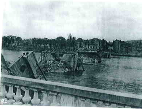
Blown Bridge at Pont a Moussen
