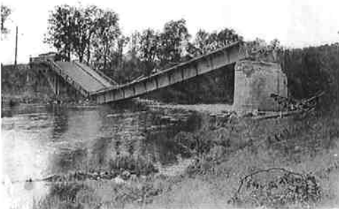
Blown Bridge at Diulard
