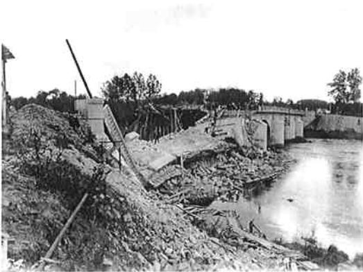
Blown Bridge at Toul
