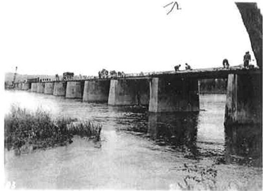
Repairing Bridge Across Moselle
