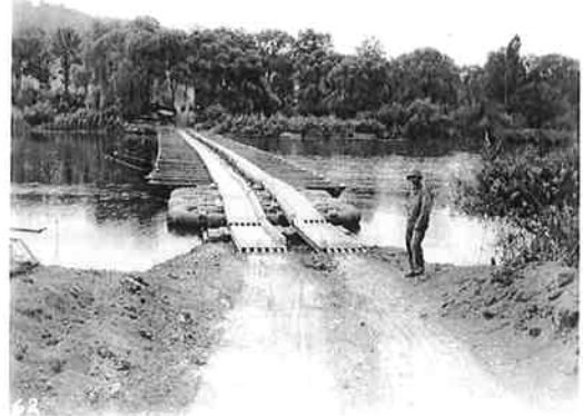
Pontoon Bridge Across Moselle
