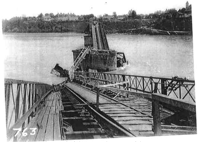
Blown bridge made passable
