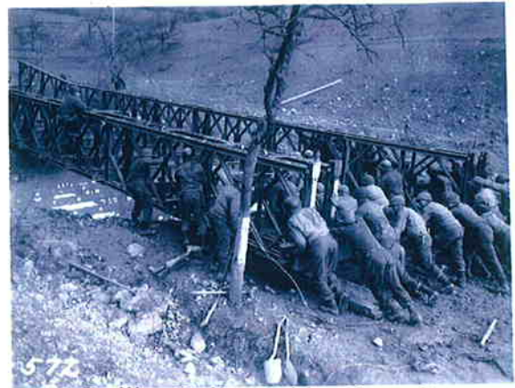
Rolling Bailey Bridge Over Crater
