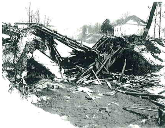
Bridge Blown, Nomeny
